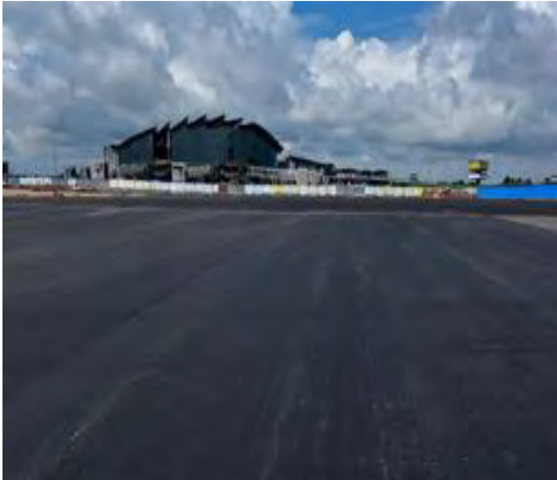
Taxiway at N-E Apron
